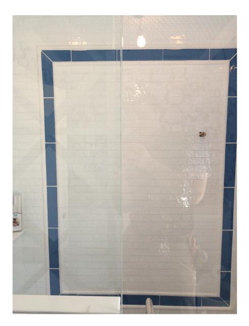
Photo represents 3/8 Clear on left side and 3/8 Low Iron on right side
