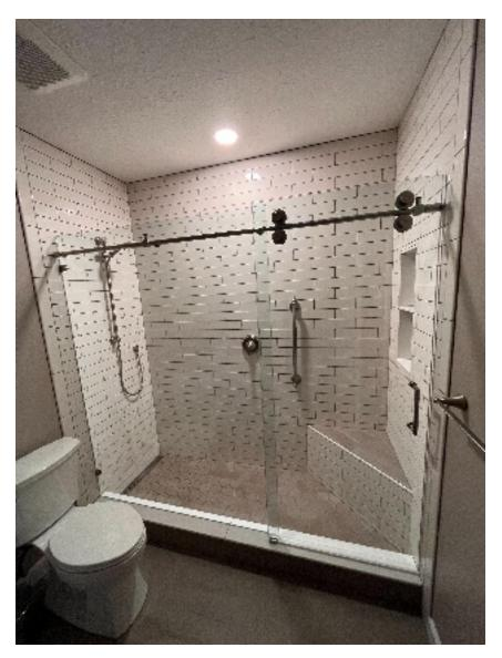
\*\*\*Notice there is no vertical metal on the sides or horizontal metal on the bottom, as you would find in box stores. While this eliminates adjustability, it adds to the customized fit and finish, clients prefer.\*\*\*
